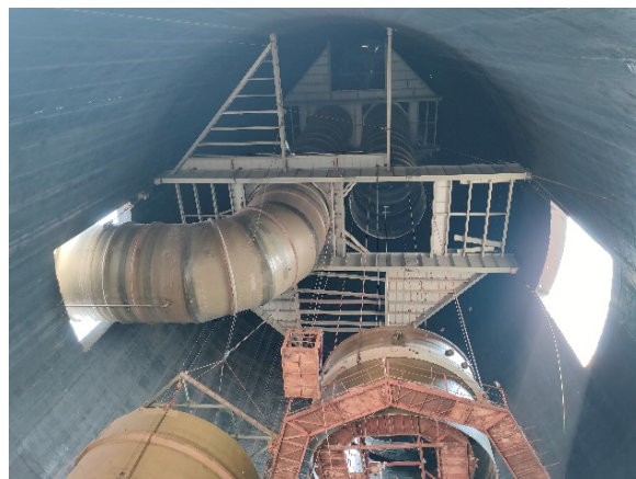
Installation activities of Flue can for 2 nd unit
