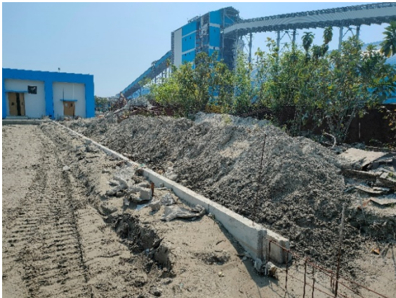
Part of drainage system is being constructed
