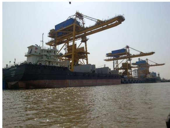
Coal Handling Procedure at Jetty Site
