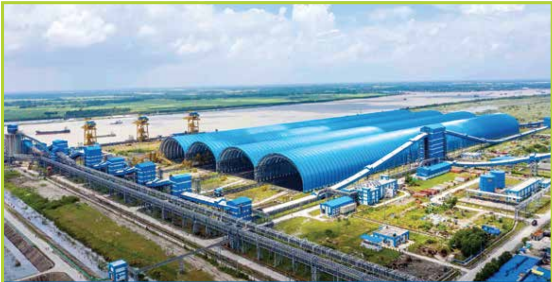
COVERED COAL STOCKYARD
