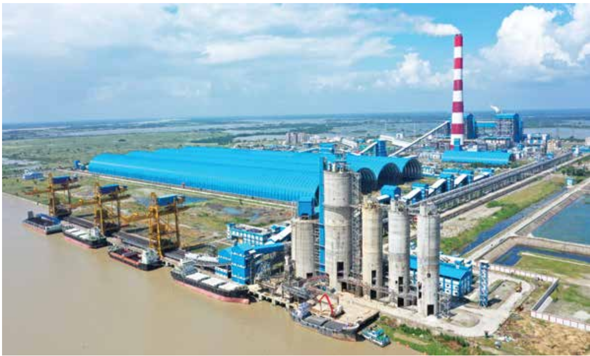
Plant Jetty and Silo
