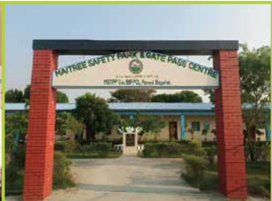
MAIN GATE OF SAFETY PARK & GATE PASS CENTRE
