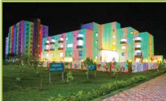
GUEST HOUSE AT PLANT SITE
