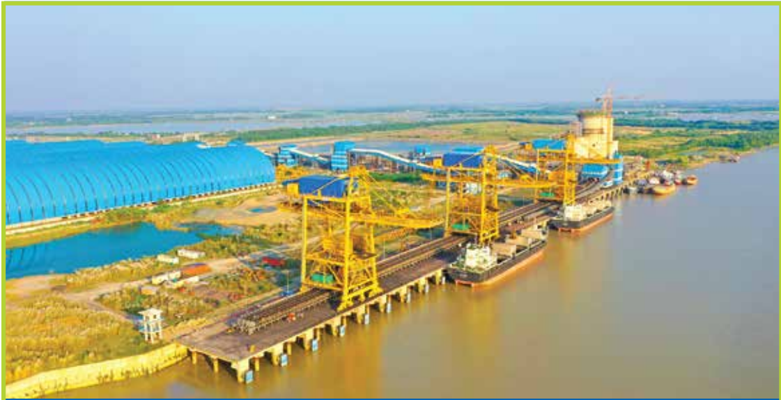
SHIP UNLOADER AT PLANT JETTY
