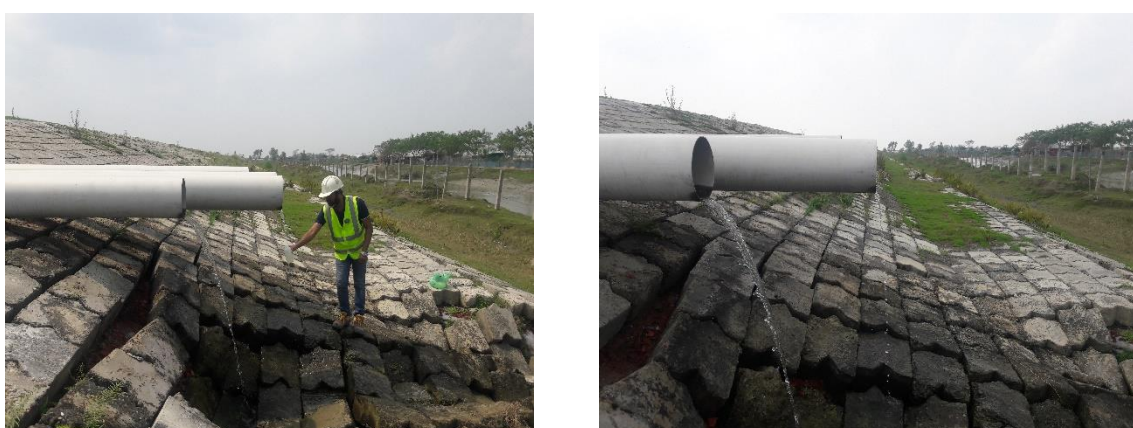
Figure 2.6: Storm Discharge Water sample collection and Discharge outlet
