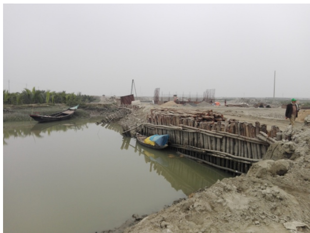
Temporary cross-dam over Maidara River restricting natural flow
