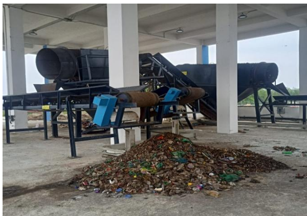
Figure 4.3: Solid Waste Management facility in MSTPP Premises
